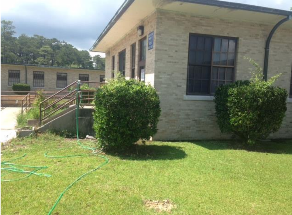
Figure 4: Site Photo: TB-3 Location
