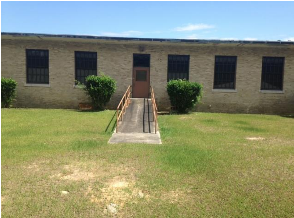
Figure 3: Site Photo: TB-2 Location
